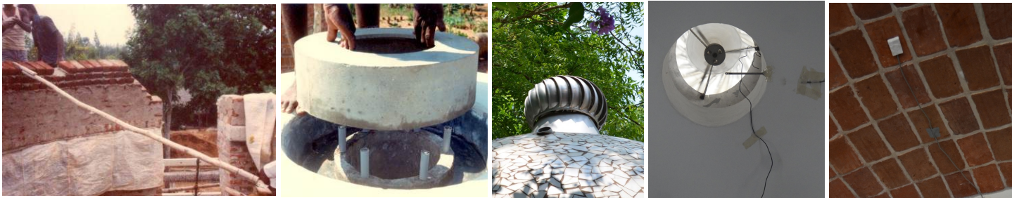
Figure 7 From the left: 1 - Dome with rotating arm under construction; 2 – Air vent opening detail on the top of the dome; 3 – Dome 2: Air vent with wind extractor; 4- Air-velocity sensor fixed in the Dome 2; 5 – Fixed surface temp sensor on the vault covered with white thermocol strip
