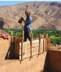
curved and continuous or organized in modules. The earth is tamped by layers inside the tapial. In cob the layers are stacked manually and can be smoothed, cut, etc. at a later stage. In this group it is also worth remembering mixed techniques, such as piled rammed earth or poured rammed earth, where a mix is poured into the formwork.
