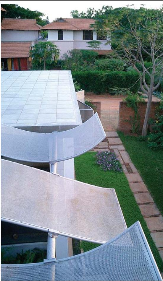
Roof shading devices
