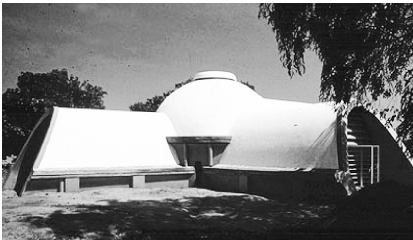
▲ Figure 9: Agni Jata Building, Auroville
