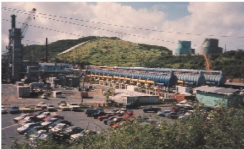
Three low-temperature MED plants on St. Thomas (VI). Each plant has a capacity of about 5,000 m 3 /d
