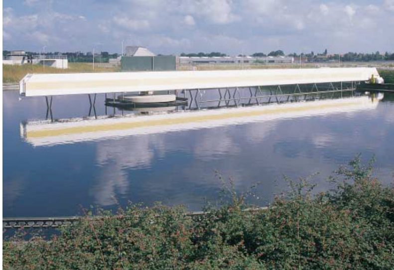
Figure H1 A clarifier as part of a large municipal waste water treatment plant.
