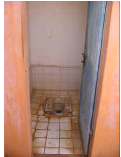
The Clean Bombay Style Toilets
