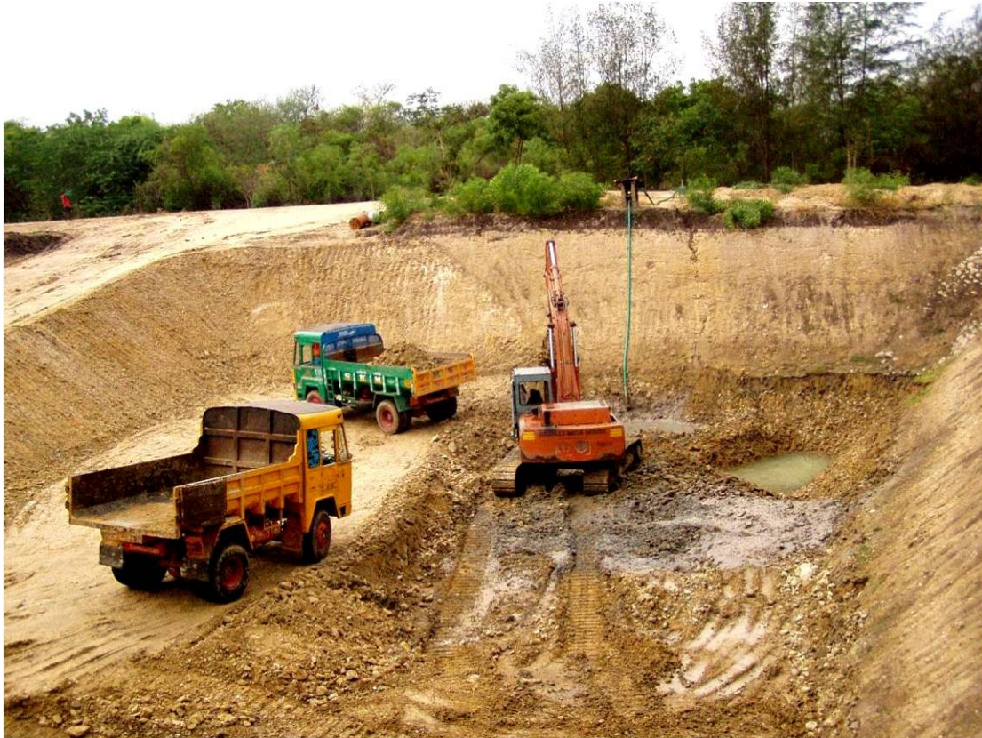
Fig 17. A trench being dug in Auroville for rainwater harvesting
