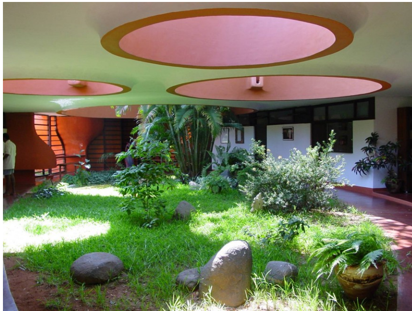
Fig 6. Efficient daylighting in an Auroville school interior
