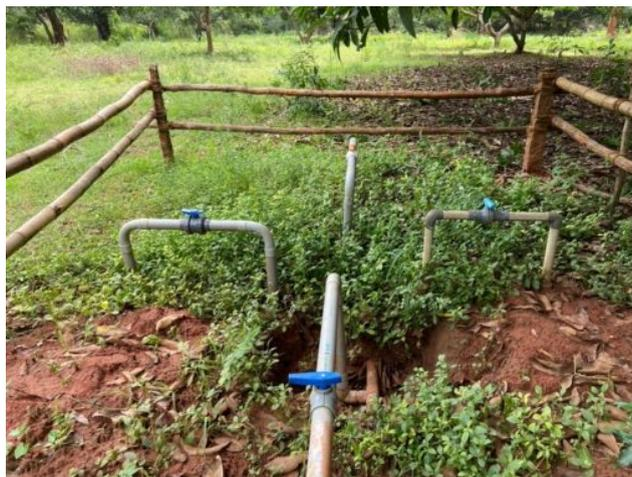
*A system that connects the Mango Borewell to the existing irrigation system in the Mango Orchard and to the entire farm*
