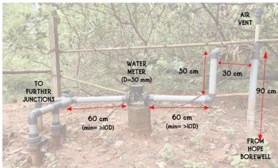
*50 mm water meter installed on Hope borewell*
