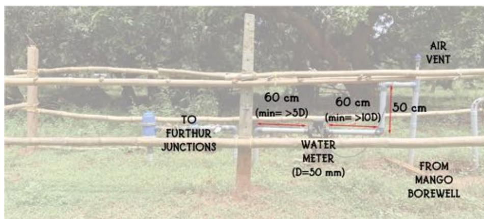
*50 mm water meter installed on Mango borewell*
