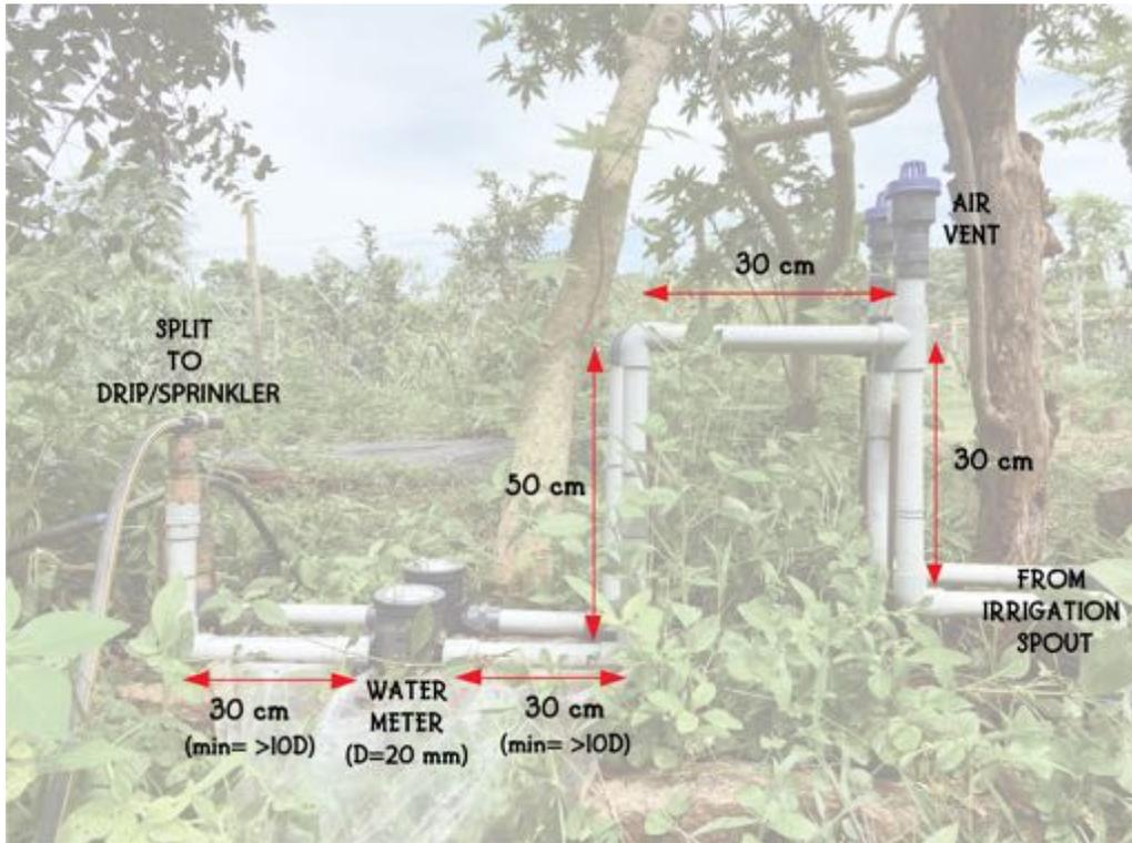
*20 mm water meter installed on cashew side of Zone B*
