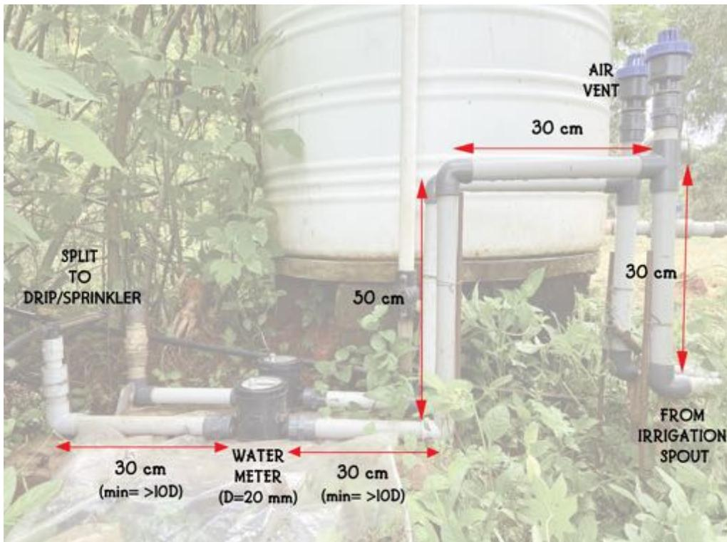
*20 mm water meter installed on coconut side of Zone B*
