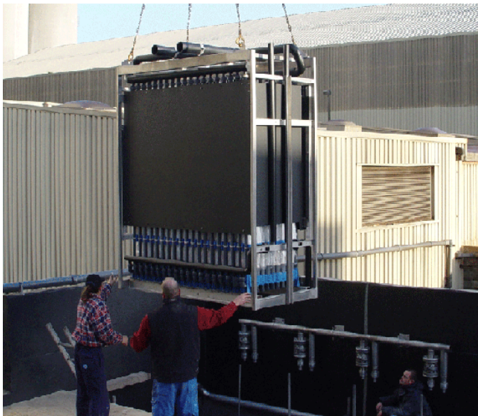
Image 6: MBR module, Koch Membrane systems “Puron”[4]
