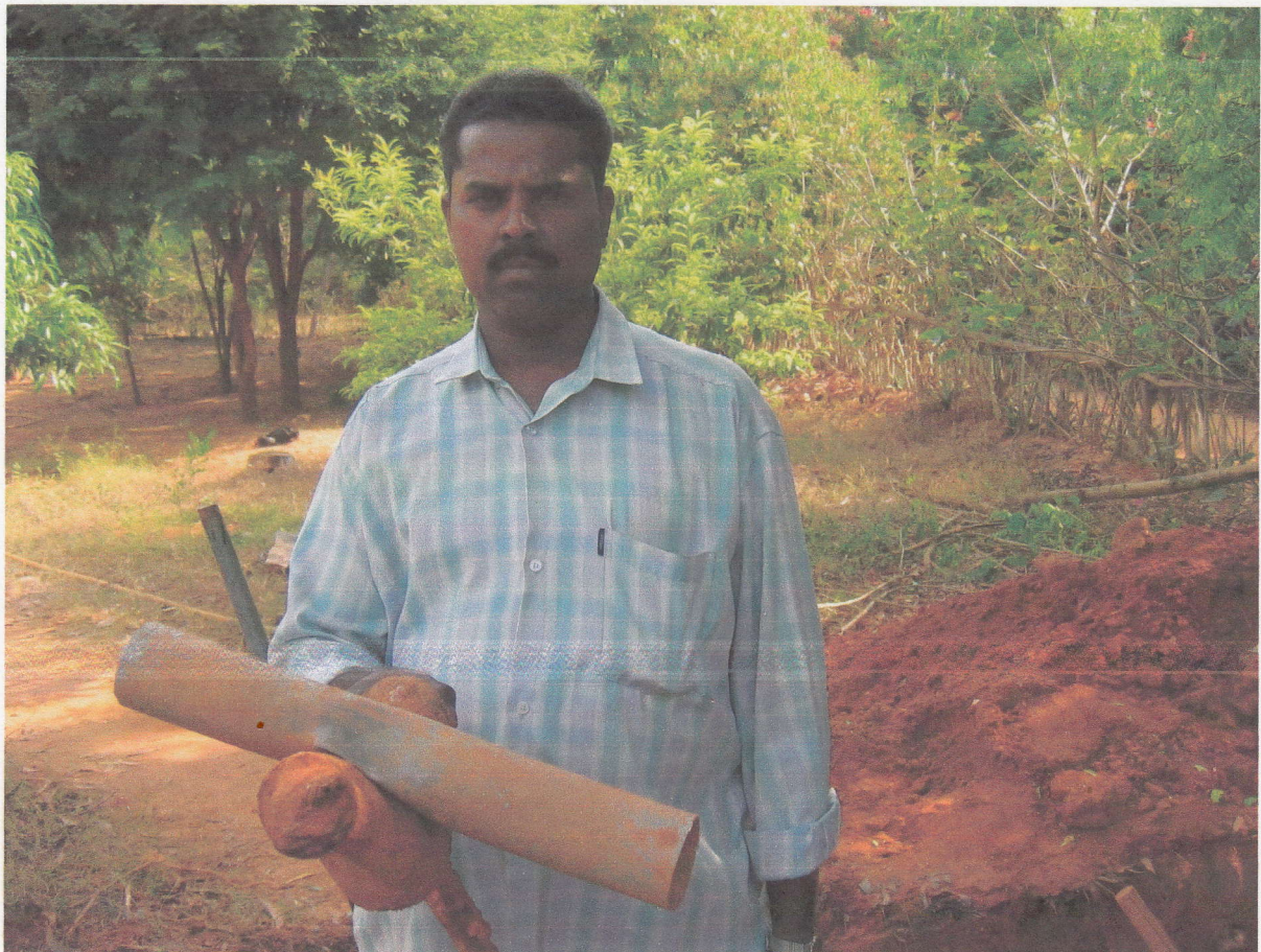
Image 29: low quality PVC pipe damaged through a Neemtree-root in Auromodele
