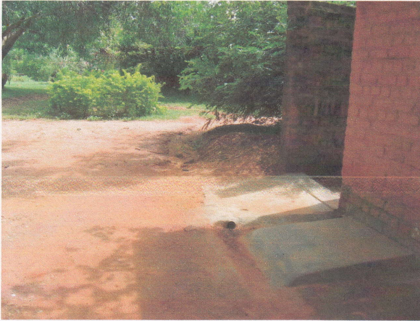
Image 26: Drainage of Storm water
