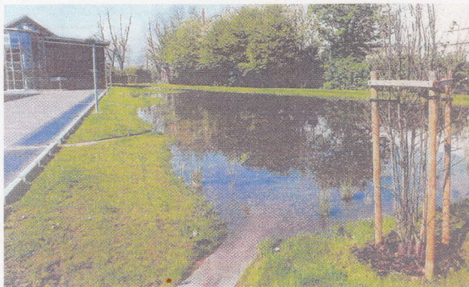
Image 50: infiltration pond next to road
