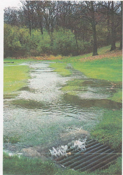
Image 17: Runoff flowing into a storm water drain
