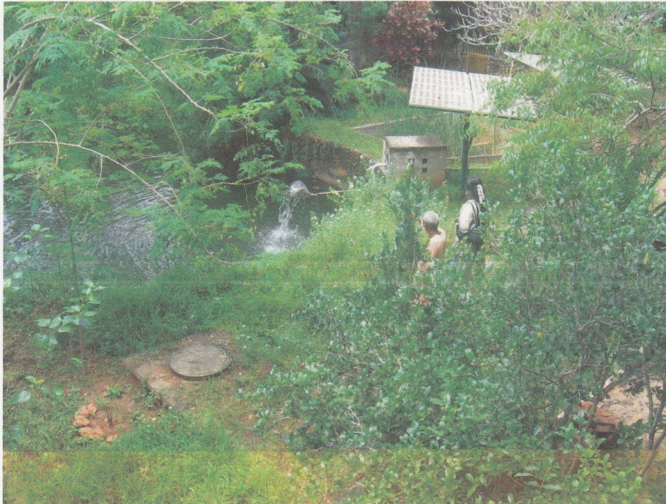
Image 13: Vikas wwt system, baffle reactor and polishing pond
