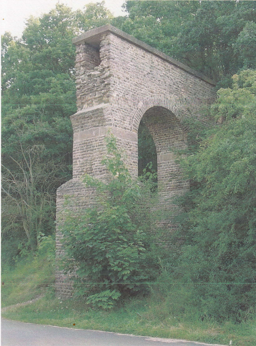
Image 47: Antique roman Aquaduct, Nettersheim Eifel, Germany
