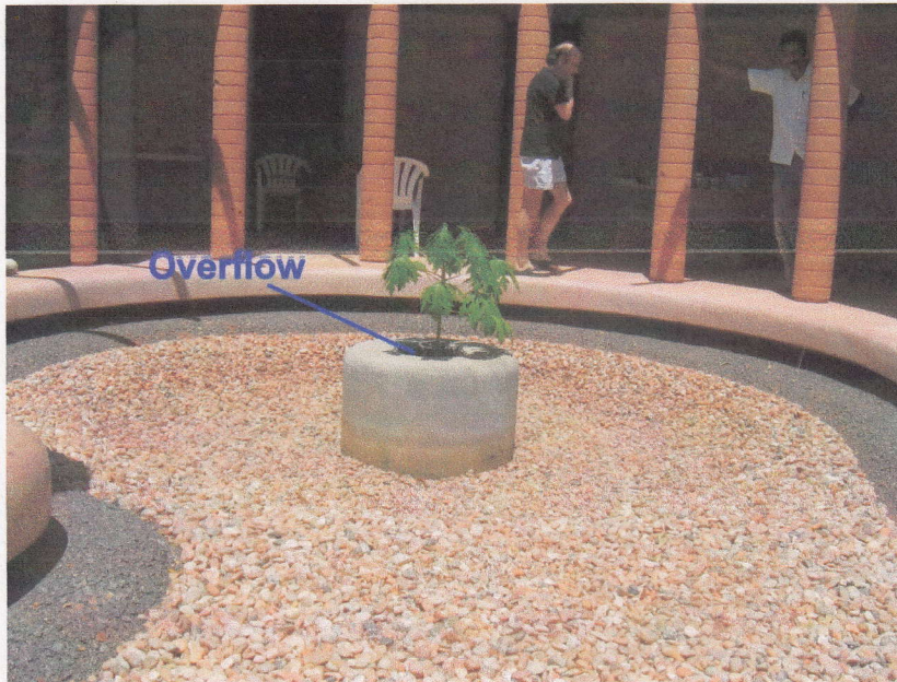
Image 24: Storm water collection pond with overflow to...
