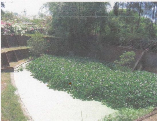
Image 11: Polishing Tank with water plants, Invocation
