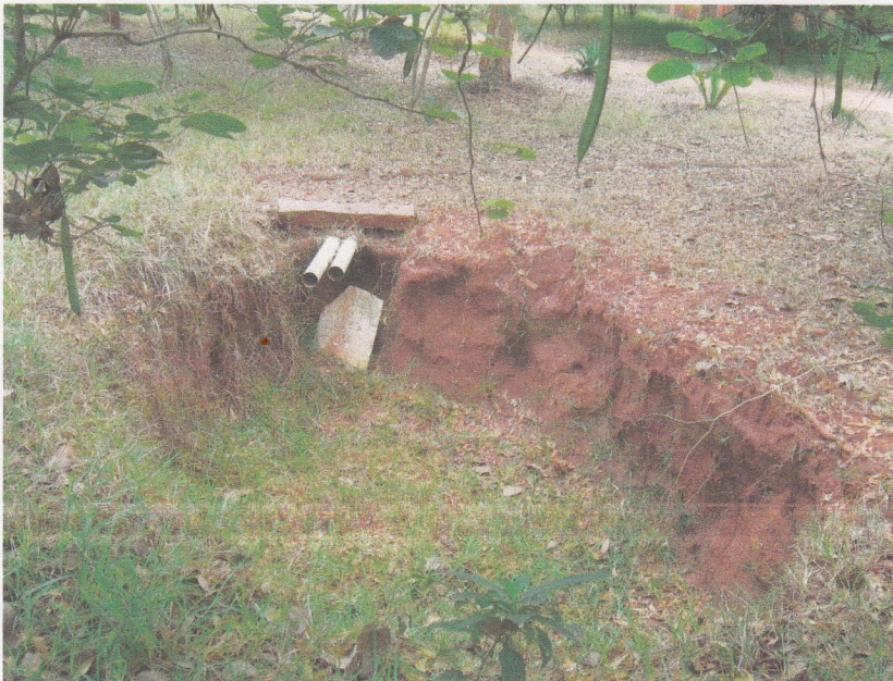
Image 21: Roof water pipe outlet
