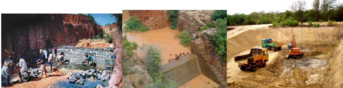
Figure 46 Check Dams and percolation ponds in Auroville
