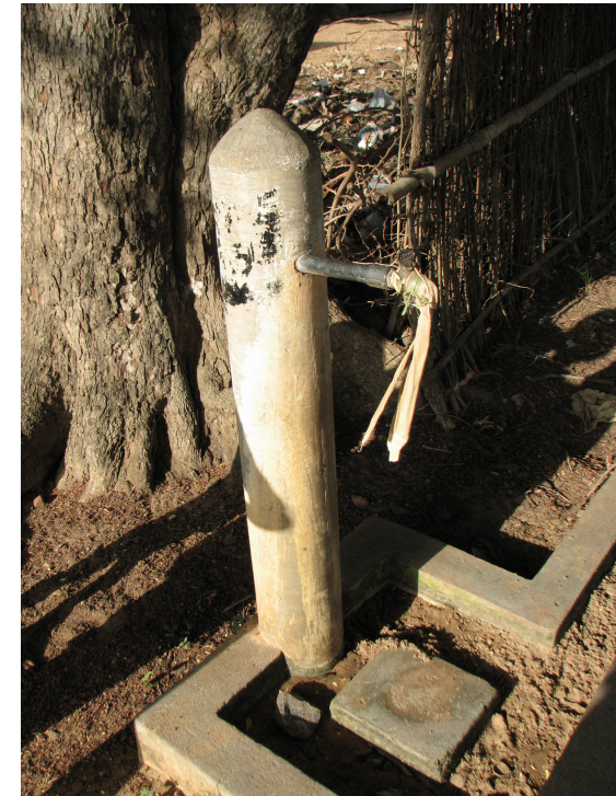
Broken taps are not replaced but improvised blocking is used leading to unhygienic situations and loss of water.
