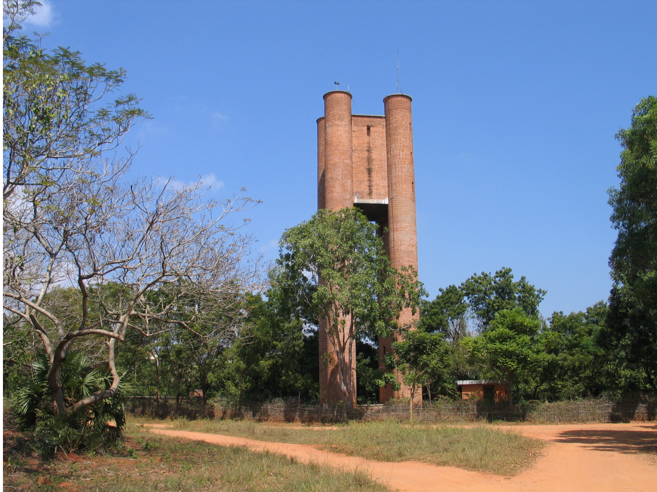
Overhead storage tank of the Invocation water supply system
