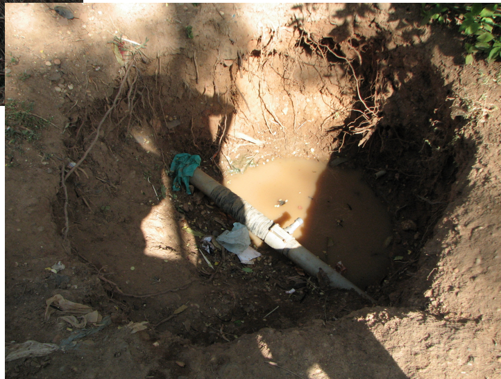
Broken taps are not replaced but improvised blocking is used leading to unhygienic situations and loss of water.
